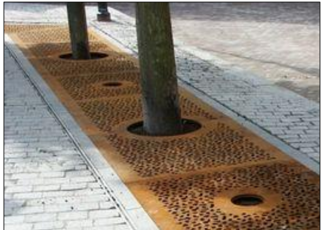
Figure 75 – Decorative Tree Grates
